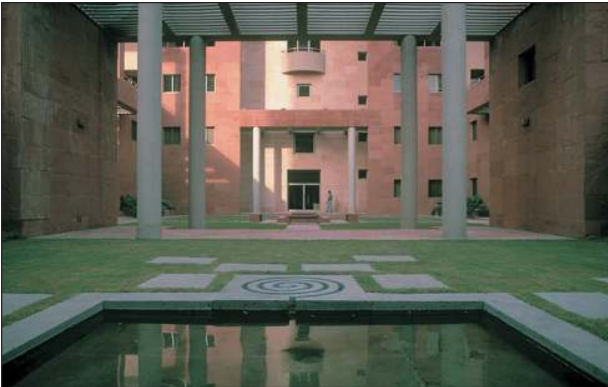
Charles Correa's design for the British Council in New Delhi is one of the architect's most well-known works
